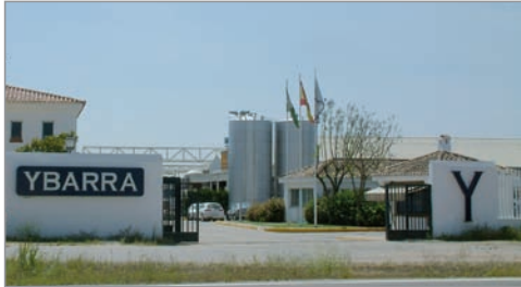
Ybarra production facility in Dos Hermanas
